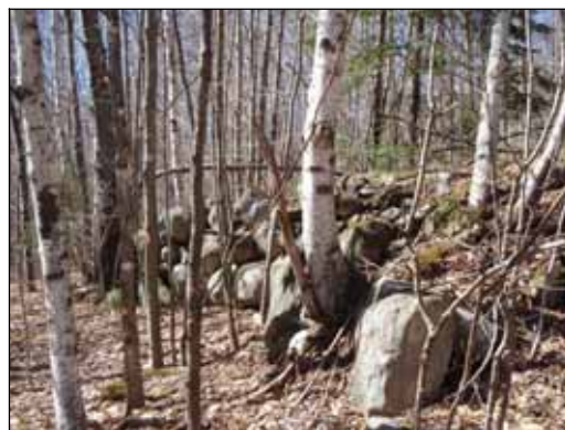
An old foundation wall
